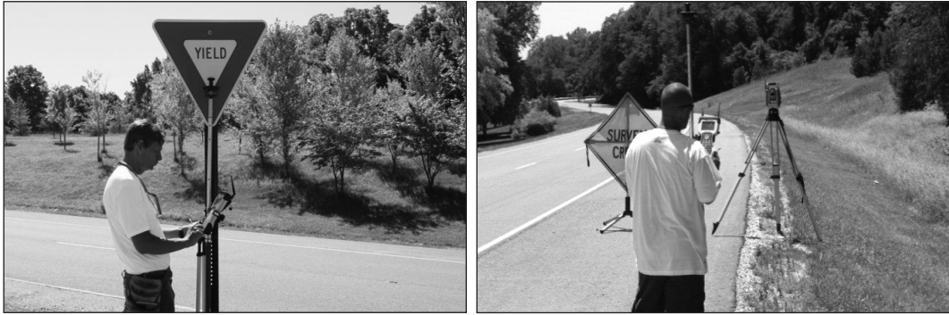
Figure 4: A Robotic Total Station Device for Data Collection
