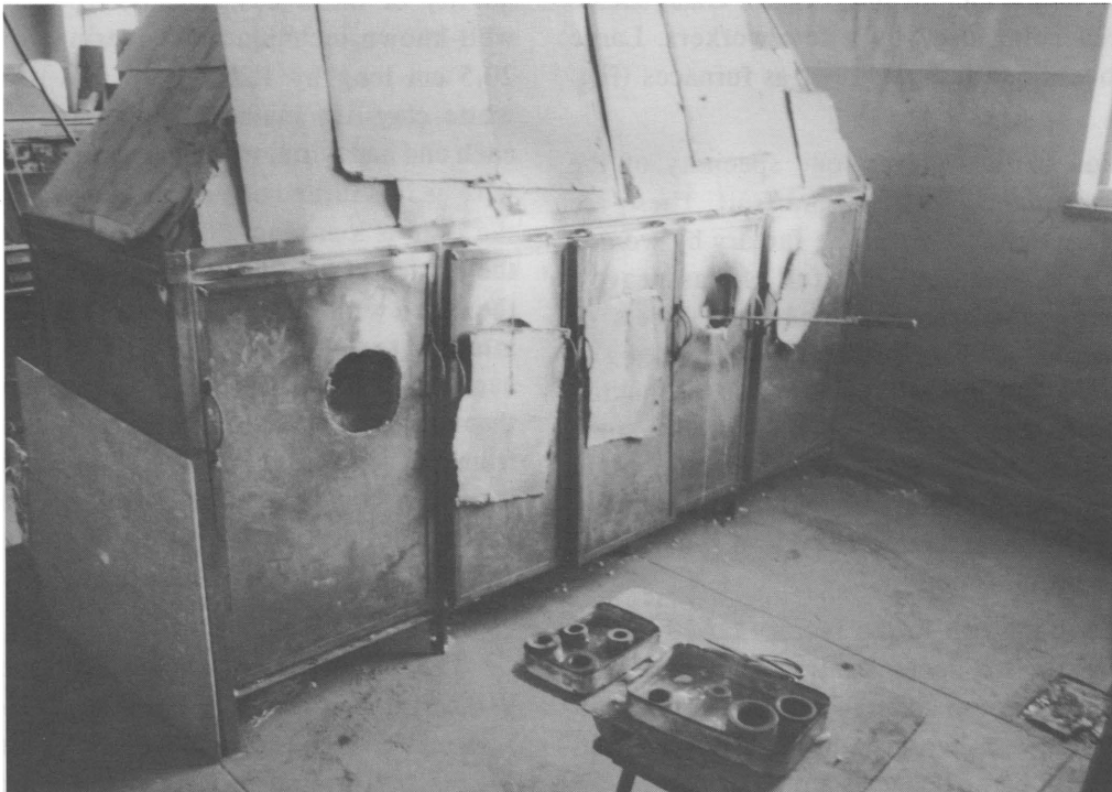
Figure 4. Gas-heated, glass-melting furnaces at the Beijing Glass Ware Factory (photo by R. Sprague).
