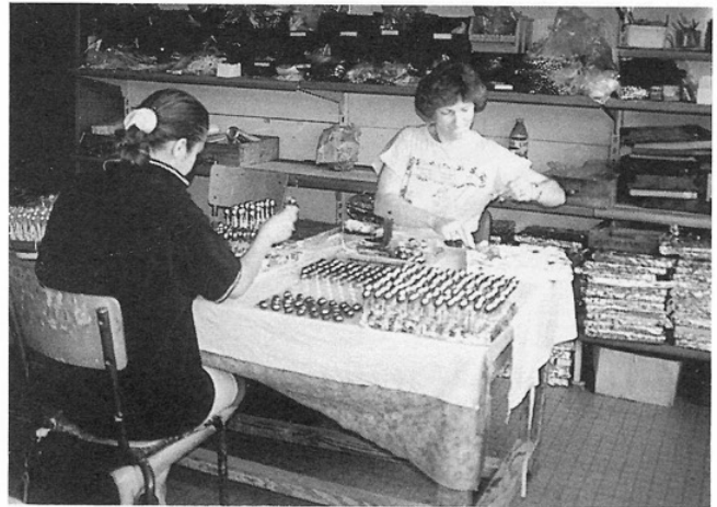
Figure 10. Technicians polishing nacreous glass beads in the workshop of Franck Alexanian.
